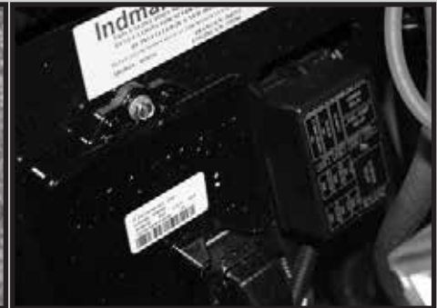
Fuse Panel - Back of Engine
