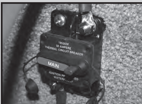
Main Dash Power-Circuit Breaker
