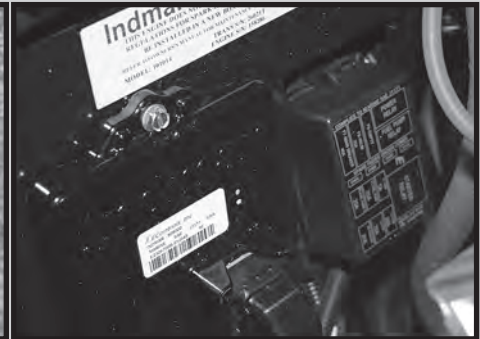
Fuse Panel - Back of Engine
