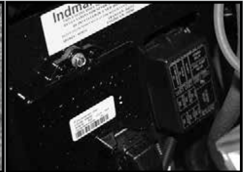
Fuse Panel - Back of Engine
