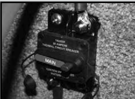
Main Dash Power-Circuit Breaker
